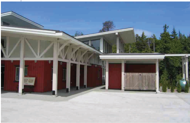
Roof or canopy structures minimize wetting of wood posts and beams.
