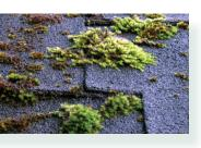
An accumulation of moss will tend to hold moisture on the roof, preventing proper drainage and accelerating the deterioration of roofing components.
