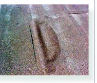
A large blister on this two-ply low-slope roof has caused the membrane to move at the seam. The membrane has split under this stress and the blister is now full of water.
