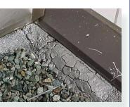
The gravel cover of this built-up low-slope roof has moved, exposing the membrane that is cracked as a result of exposure to sun and weather, and exposing the underlying roofing felts. The roof can be expected to deteriorate quickly, and may already have failed at this location.
