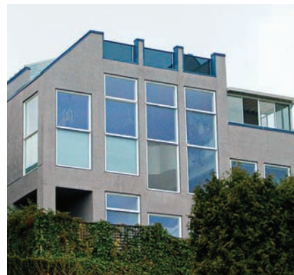
These windows are very exposed to wind-driven rain. Water resistant products and installation methods must be used.
