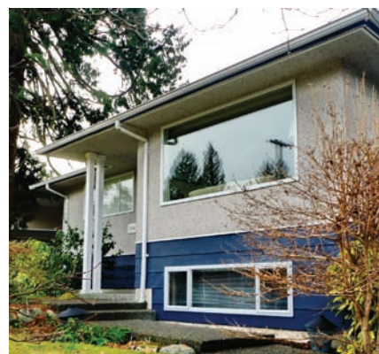
The upper windows on this home are protected by overhangs, allowing for more options when selecting products or evaluating installation methods.
